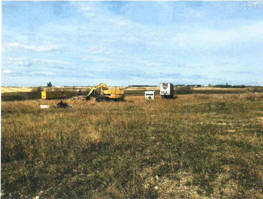
Photo 13: Looking southwest from the northern former gravel extraction site. Showing the excavator, trailer, and RV unit.
