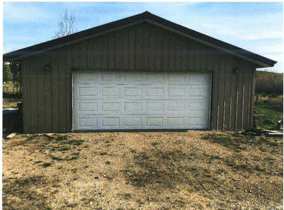
Photo 24: Single door garage/shed located east of the mobile home
