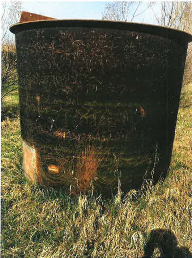
Photo 25: Fibre glass above ground storage tank located south of the garage buildings. No leaks, stains or stressed vegetation were noted around the tank during the Site visit.
