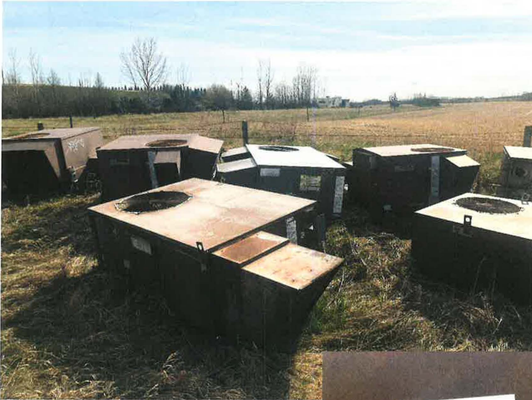
Photo 11: Collection of old heating and heating/cooling units. No staining or associated liquids were found around the units.
