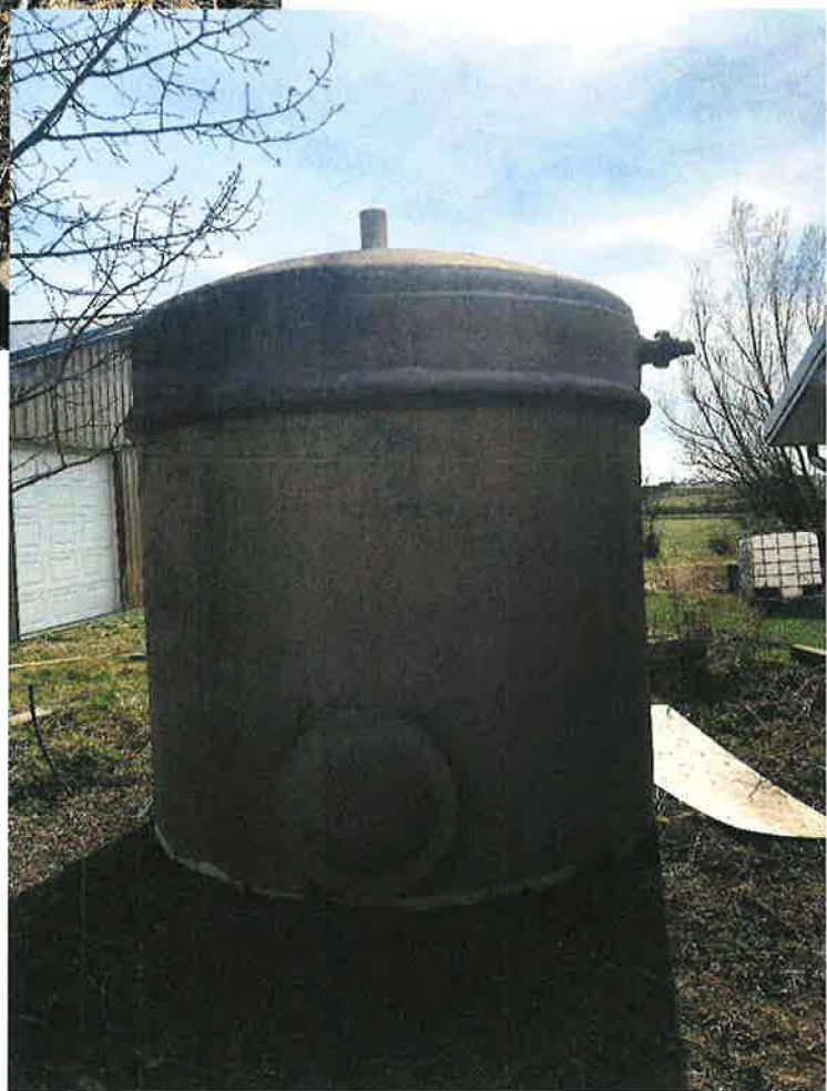
Photo 22: Water storage tank behind the double door garage. No leaks or staining around the tank was present.
