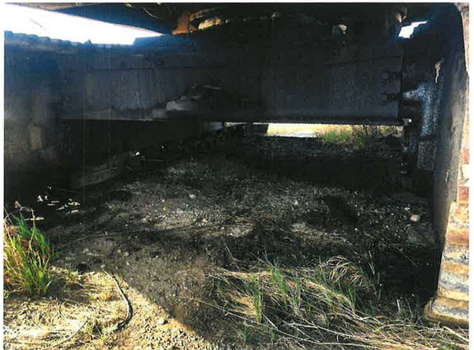
Photo 14: Ground surface under the excavator unit is relatively clean with the exception of a small spot to the front shown in Photo 15 below.
