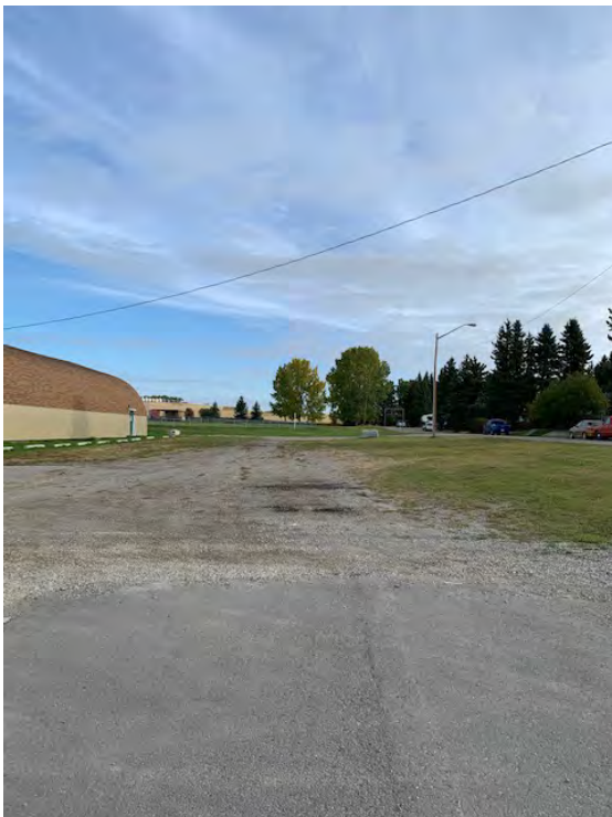
Hall Parking area looking north
