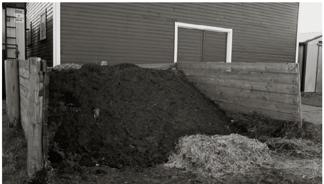
Figure 8. Three-walled structure contains the manure and can easily be covered with a tarp.
