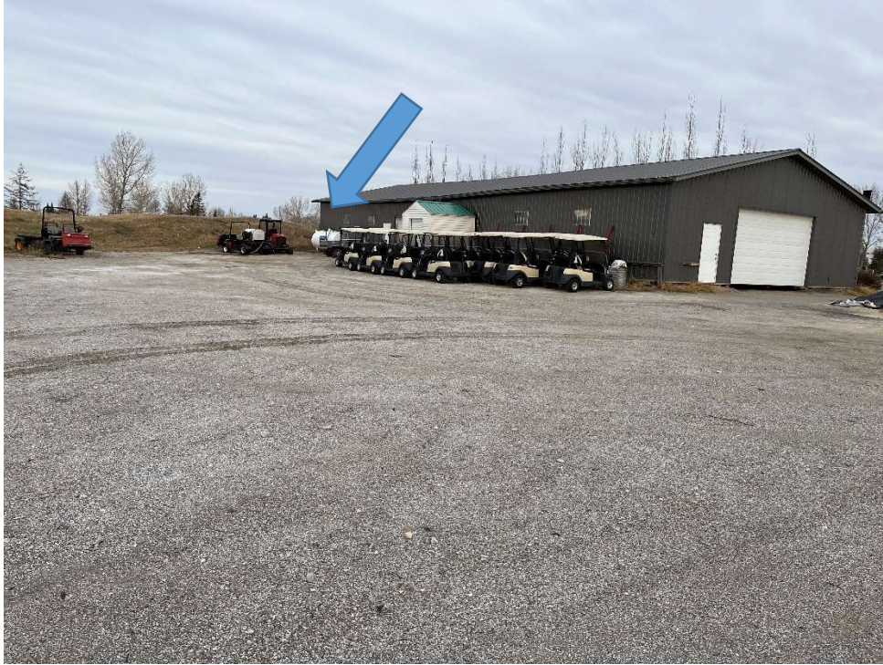
27. View of the AST (arrow) located on the west side of the battery charging building; photograph taken facing northeast.
