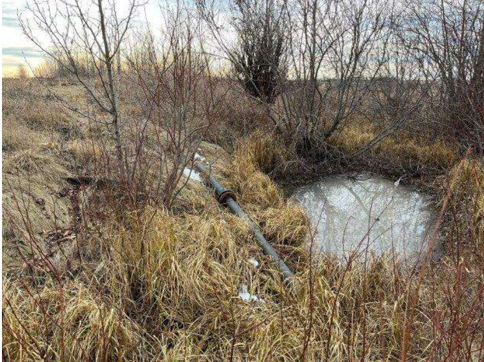
16. View facing south west of the water line that runs from the pump house on Location 2 to the southern property line along the western property boundary.
