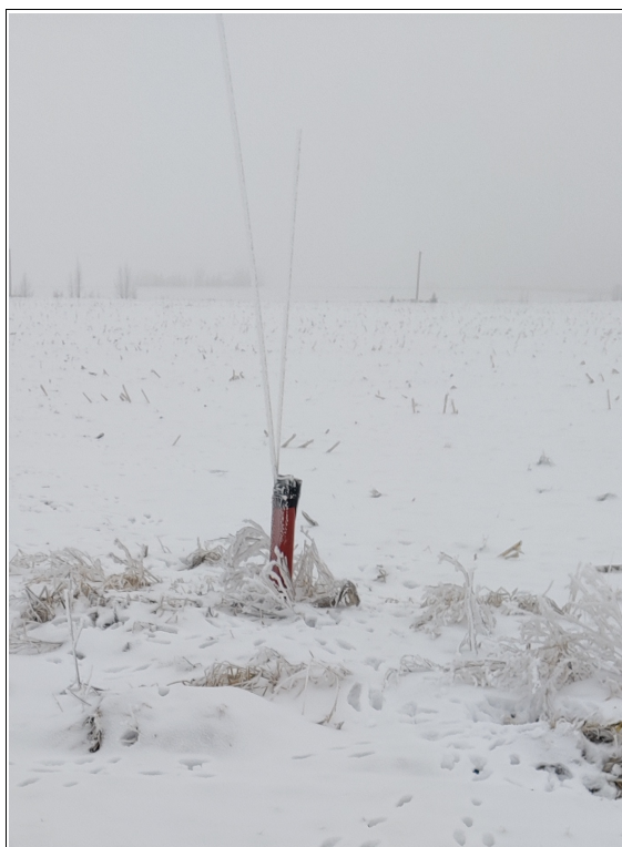
Illustration 1: “monitoring well” located with 07-03-033-01 W5 (see Figure 1-3 for location)
