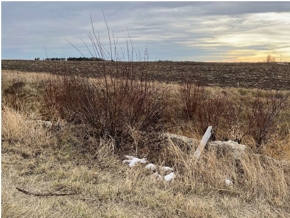
30. View of what appears to be a former concrete retaining wall, north of the Project Site; photograph taken facing southeast.
