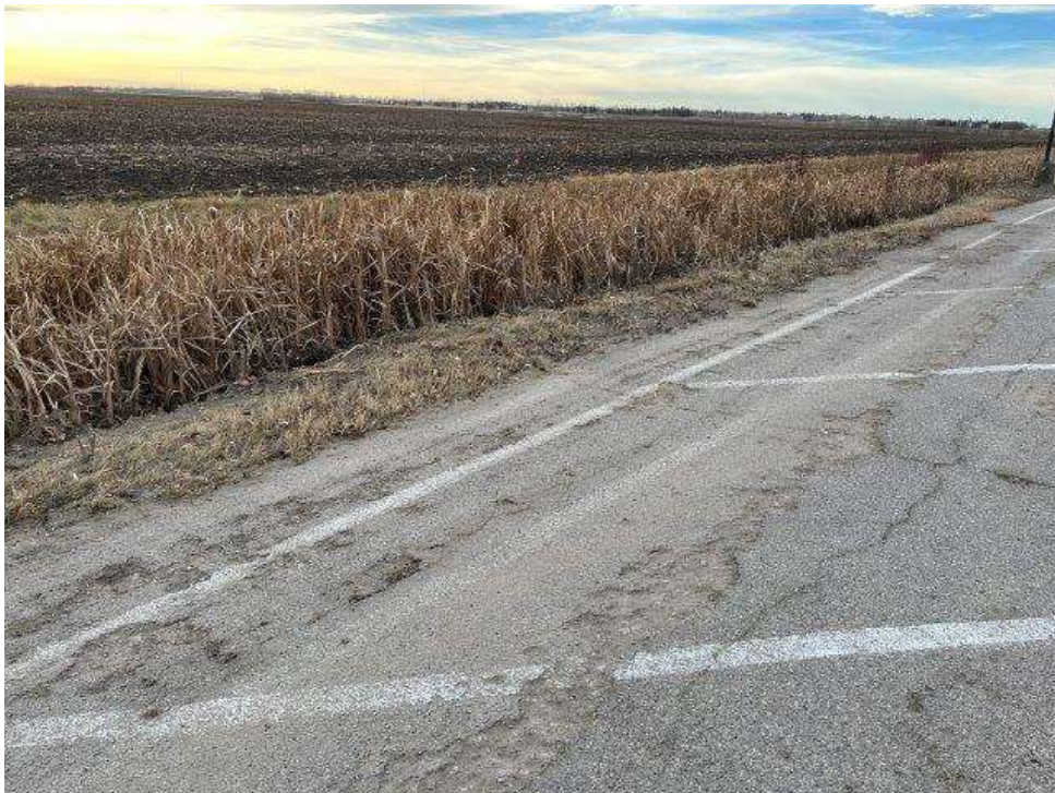
14. View to the south along the northern Project Site boundary. The change in vegetation type is clear and indicates the location of the drainage ditch.
