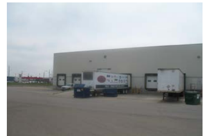
Examples of parking and loading area placement in a Distribution Centre Development Typology.
