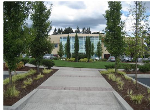
Example of well-defined building entrance
