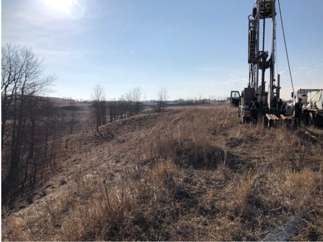
Photograph 1 – Borehole BH21-01 Location
