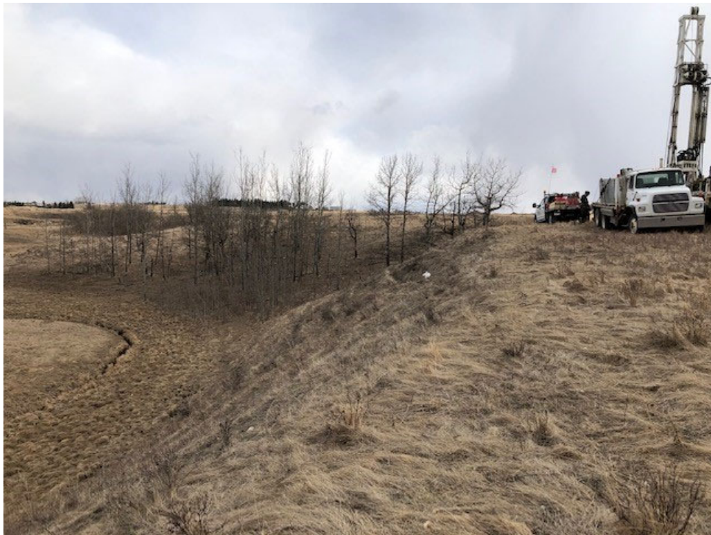
Photograph 2 – Borehole BH21-02 Location
