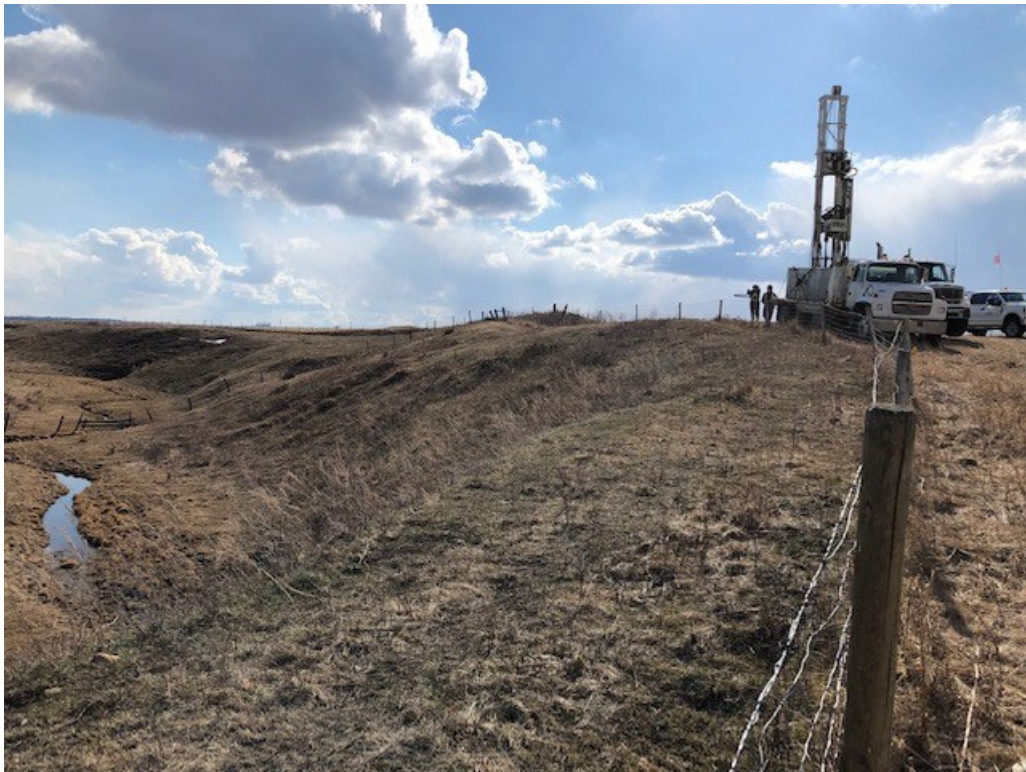
Photograph 4 – Ravine located at south end of development adjacent to Borehole BH21-03 Location
