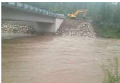
Big Prairie Bridge site on June 21, 2013
