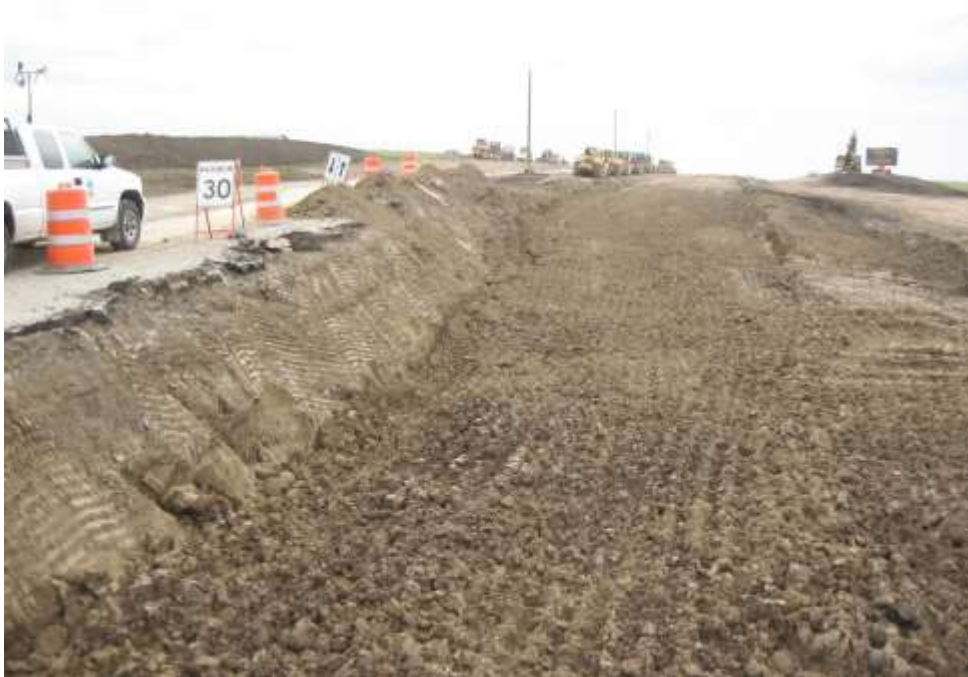
CONSTRUCTION WORK ON ACME ROAD
